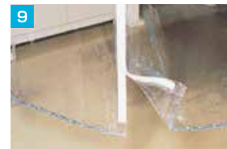
9 Chain Chain to reduce curtain movement.
